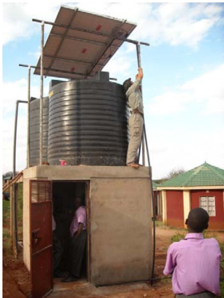
Fig 7. Completed power house, water tank, and solar panel structure.
