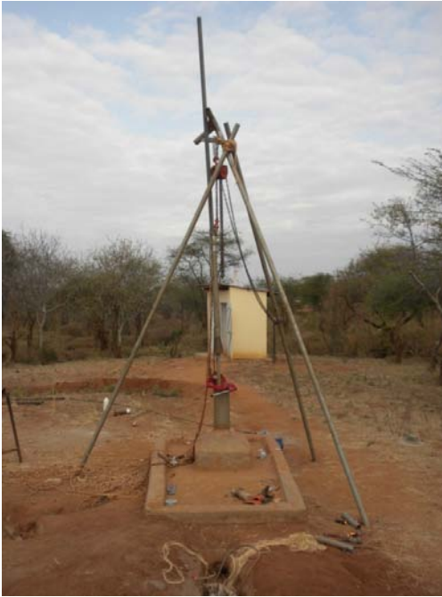
Fig. 6. The tripod, chain hoist, and rocket holding the first pipe segment out of the borehole.
