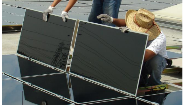
Figure 2: Thin film PV modules being installed
