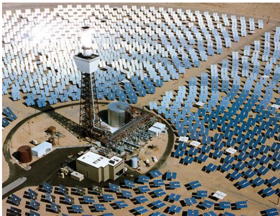
Figure 4: A Luz Power Tower 550, made by BrightSource Energy
